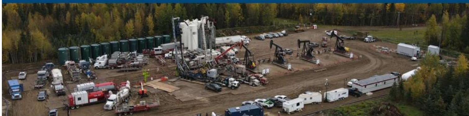
Fracture completion operations at InPlay 7 well pad in Pembina Region (October 2025)
